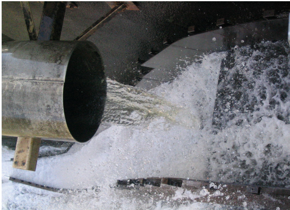
Figure 9. Downstream Fish Bypass on the Ellsworth Dam:
