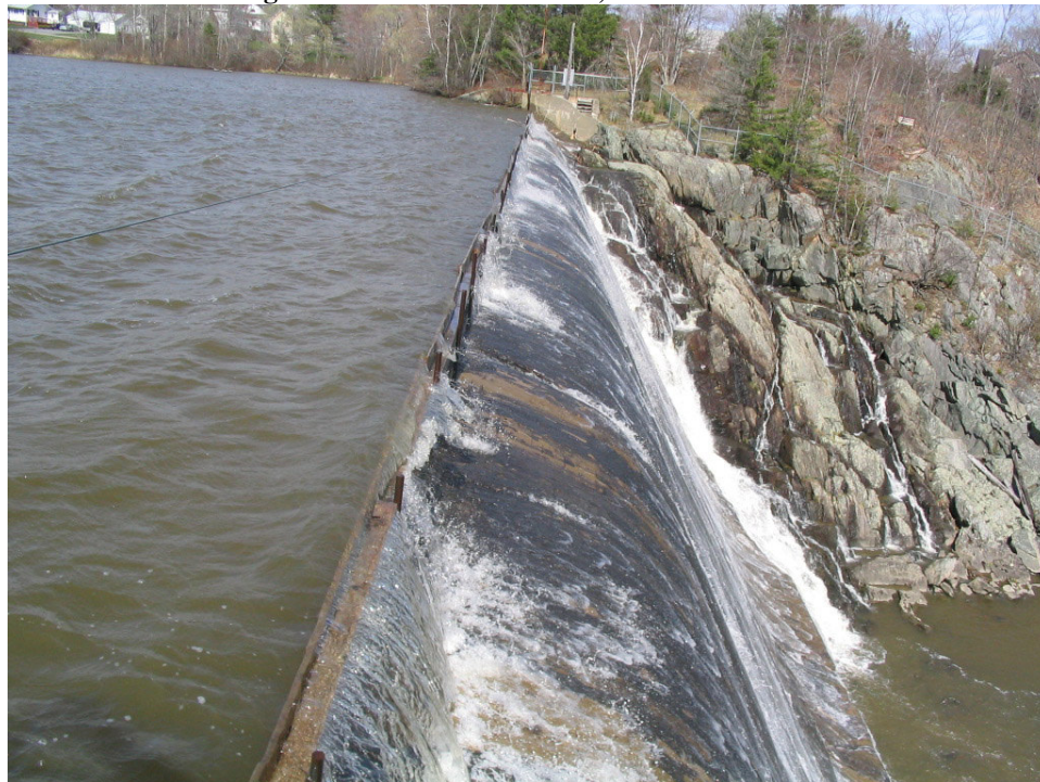
Figure 7. The Ellsworth Dam, a View from Above:
