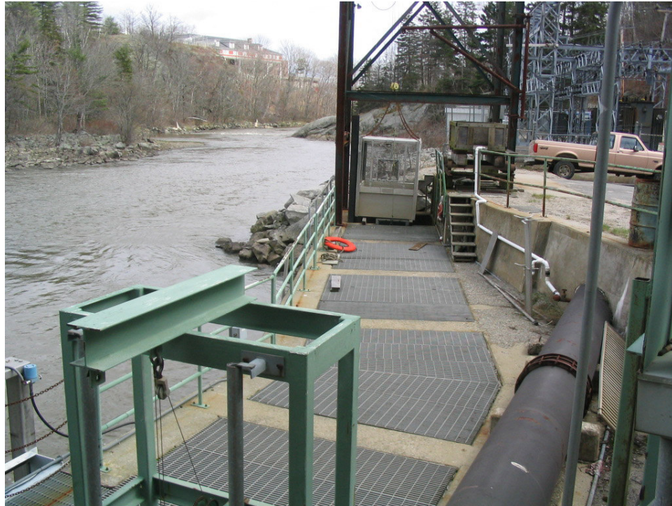
Figure 5. A Trap and Truck Facility at the Ellsworth Dam:
