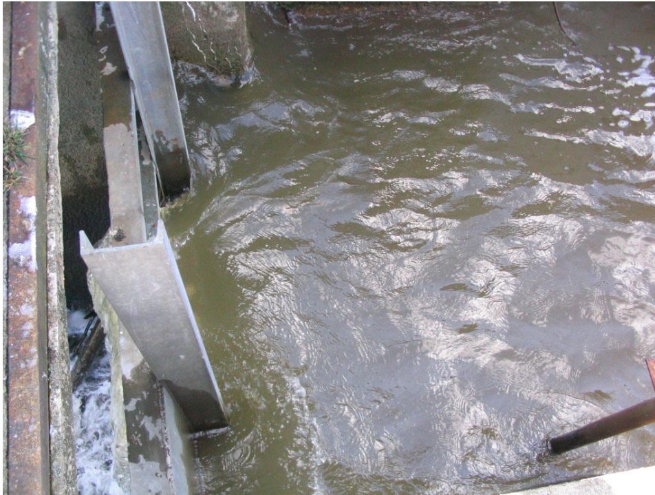
Figure 8. Entry Point for Downstream Bypass on the Ellsworth Dam:
